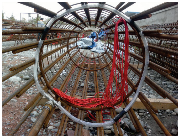
Figure 2 The embedded grouting pipe around pile foundation of 3c2
