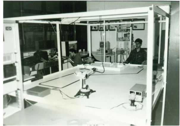
Figure 9. The experimental setup for control of a physical object using EEG signals, 1988.
