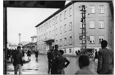
FIG. 6 PTT BUILDING SL. 6. PTT ZGRADA
