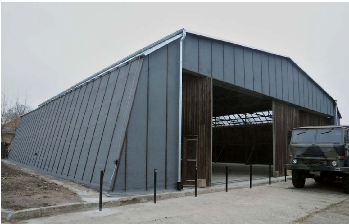
Figure 15. Immaculate restored type In specimen in Krakow. The eaves gutter with drainpipe and lightning rod are modern, but "accessories" that make sense
