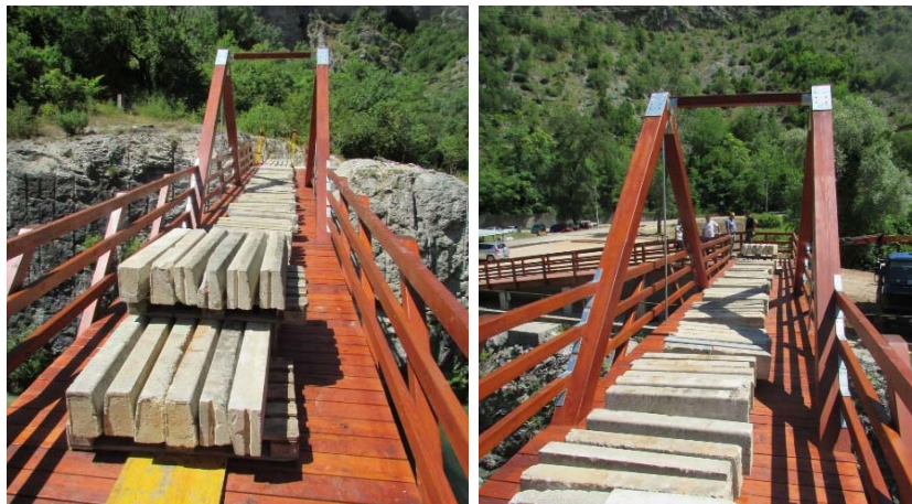
Figure 14. Test load on the bridge
