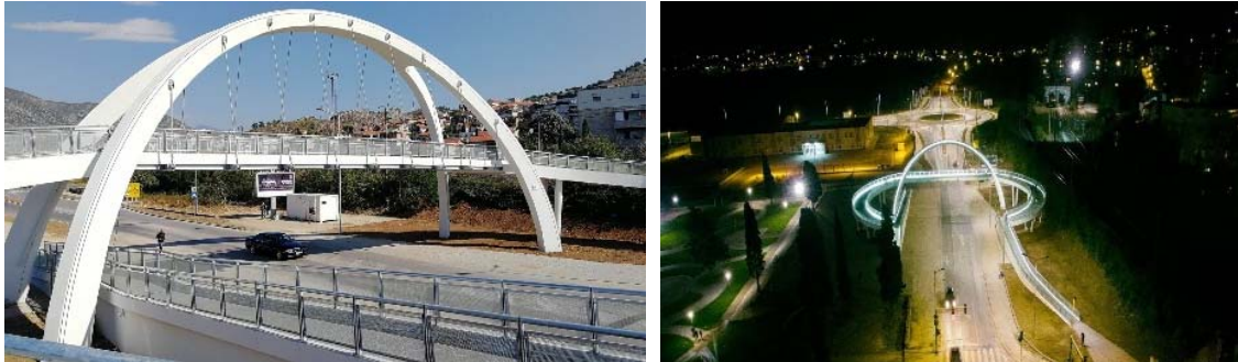
Figure 8. Pedestrian bridge at the northern entrance to the City of Mostar
