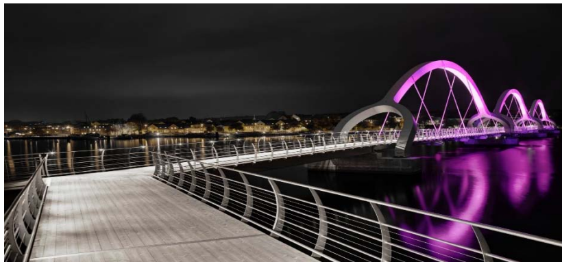
Figure 2. Sölvesborg Bridge, Ljusarkitektur, Sweden
