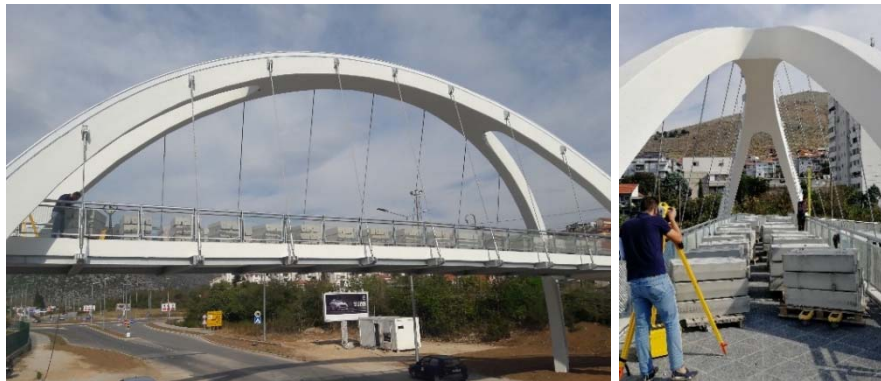
Figure 9. Test load on the bridge
