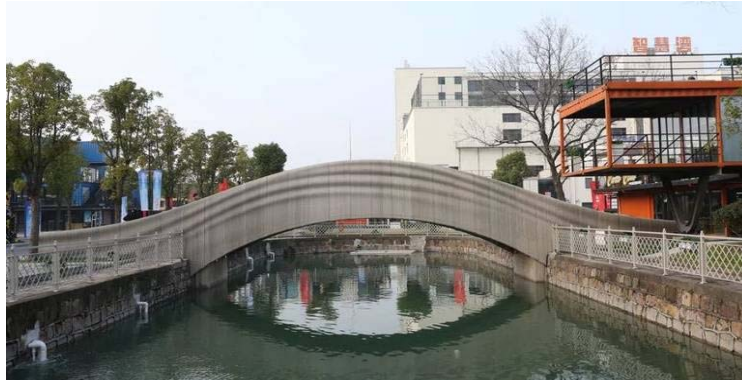
Figure 5. Pedestrian Bridge Shanghai, China - 3D print
