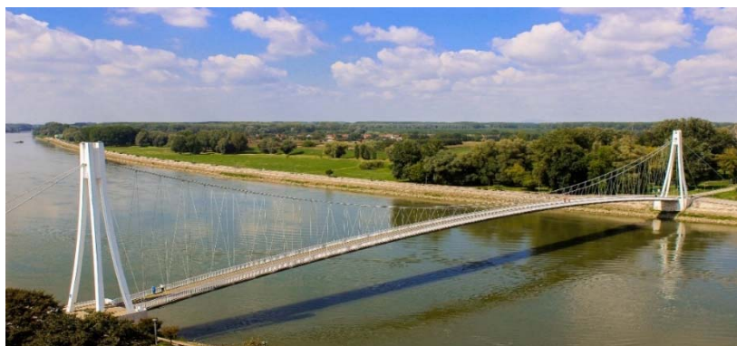
Figure 6. Pedestrian bridge (White Bridge, Bridge of Youth), Osijek, Croatia
