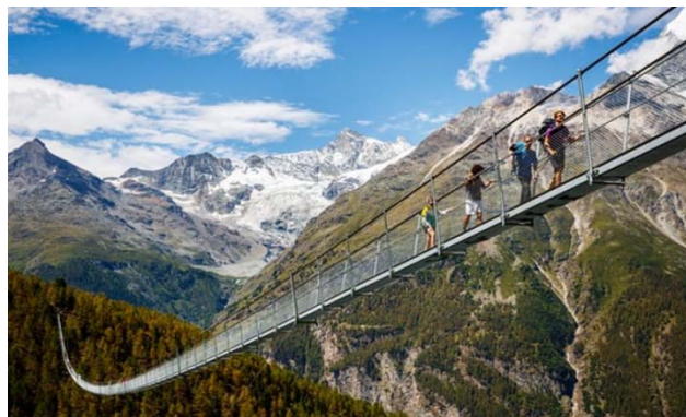
Figure 1. Charles Kuonen Suspension Bridge, Switzerland
