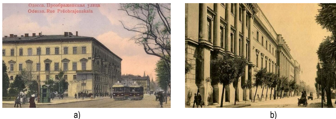
Figure 2 a) Grain shops (House of Papudovs) built in the 1st half of the 19th century [17] and b) Grain shops that were later converted to Saban barracks in 1827 [18]
