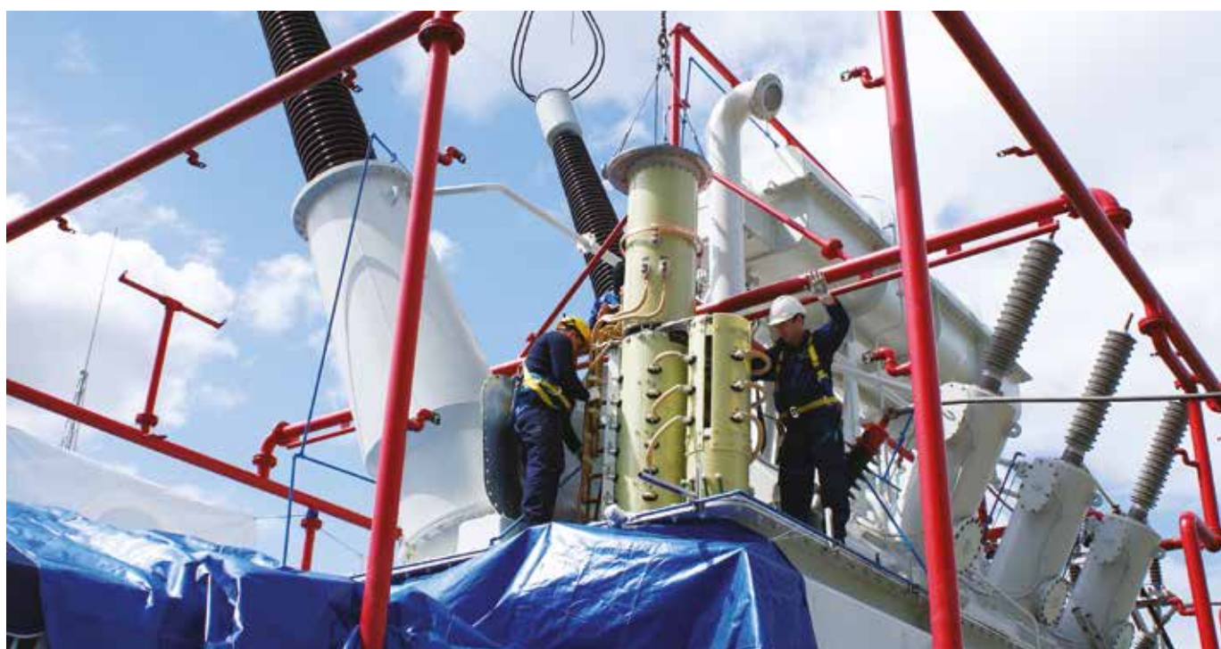
Figure 4. OLTC replacement in a transformer on site
