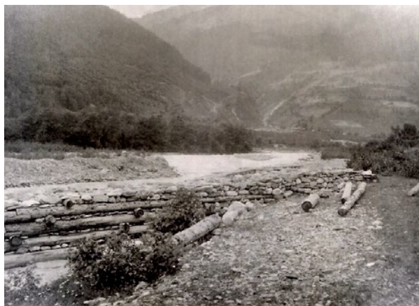
Figure 12 Destroyed dams, Möll-valley around 1882. Source: KLA, Bildarchiv Ferdinand v. Staudenheim Kärntens Wildbäche 1886, kleine Kasette Nr. 88.
