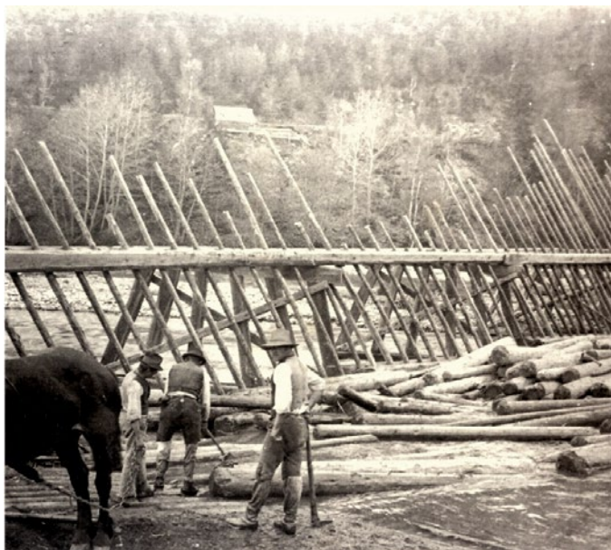
Figure 7 Wooden boom to stop the floated timber, Möll-valley (Mölltal) at the beginning of the 20 th century. Source: Archive Forest enterprise Lainach
