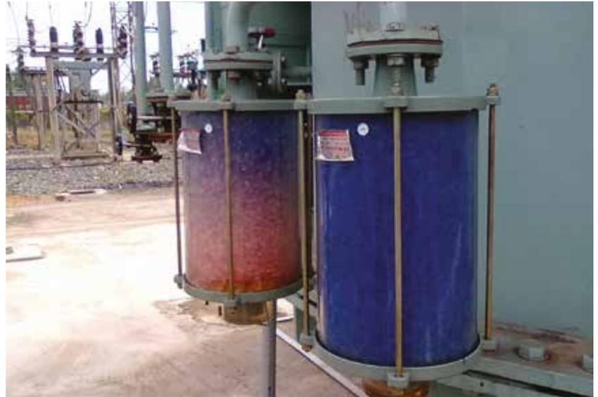
Figure 1. Colour change due to saturation of the silica gel; the breather on the right is still able to absorb water; the breather on the left is saturated with water and requires maintenance
