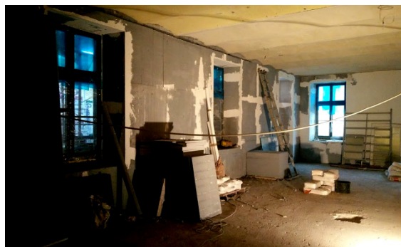
Fig. 4 General refurbishment of the tenement house, Cracow 14.04.2016
