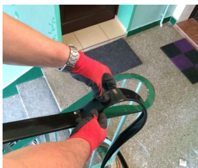
Fig. 1 Installation of rubber overlays on the handrail in the staircase
