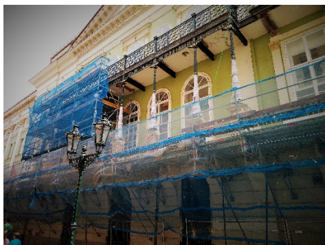
Fig. 3 Refurbishment of balconies in a historic tenement house, Prague 23.05.2016
