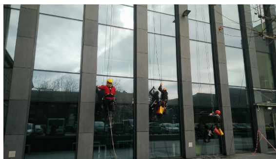
Fig. 2 Cleaning glazed surfaces, 02.2017, Cracow
