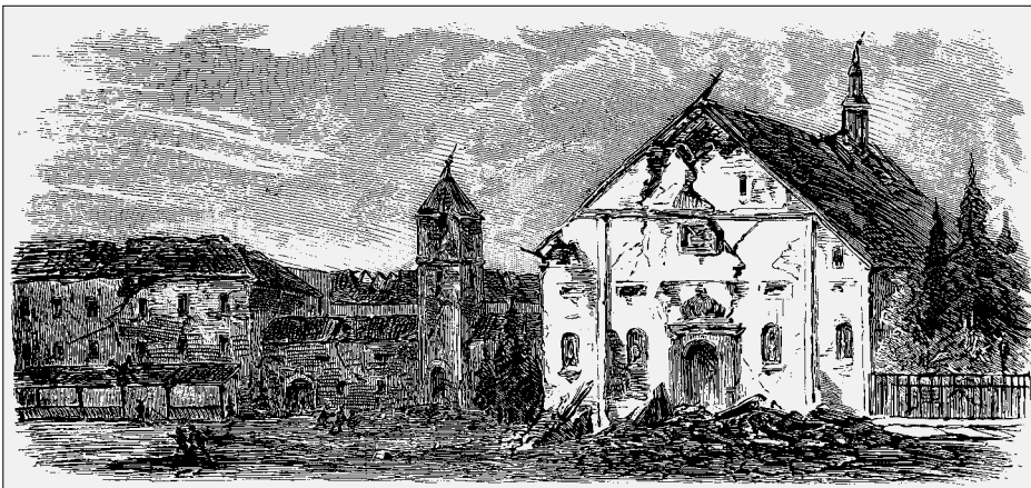
FIG. 6 MAIN FACADE OF THE GENERAL COMMAND BUILDING AND THE CHURCH OF ST. CATHERINE DAMAGED IN THE EARTHQUAKE, ACCORDING TO THE GRAPHIC BY J. SMUTNYJA
