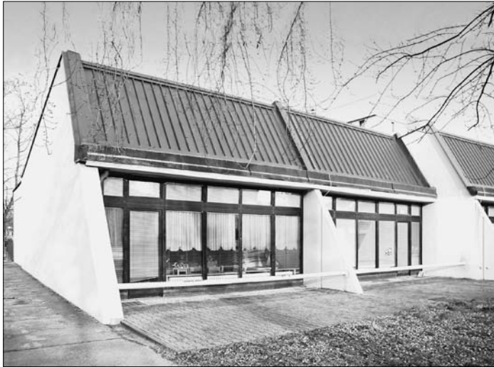
FIG. 4 CLASSROOM WITH ORIGINAL WINDOWS (A) SL. 4. UČIONICA S IZVORNIM PROZORIMA (A)
