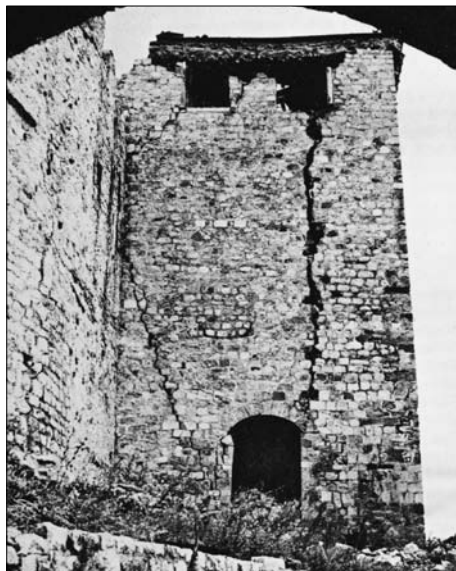
SL. 2. OŠTECENA KULA BALSICA U STAROM GRADU ULCINJU FIG. 2 DAMAGED THE BALSIC TOWER IN THE OLD TOWN ULCINIJ
