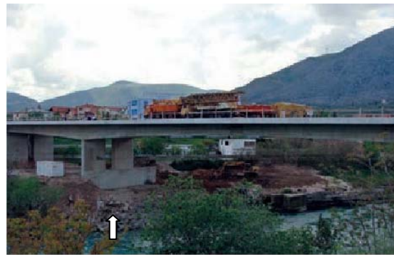
Figure 9. Protection of the right bank near the river pier of the New Bridge on Neretva [11]
