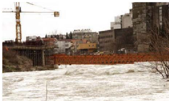
Figure 7. Construction site of the New Bridge in 2010 [11]
