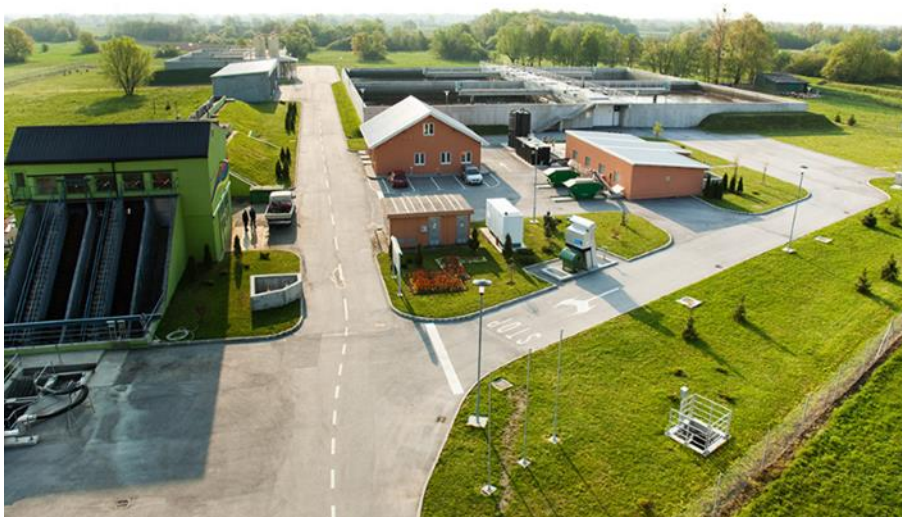
Fig. 2. Biological wastewater treatment plant in the city of Koprivnica (source: www.kcvode.hr )
