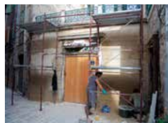
36 Projekt 45: stanje uličnog zida u tijeku radova Project 45: condition of street wall during restoration
