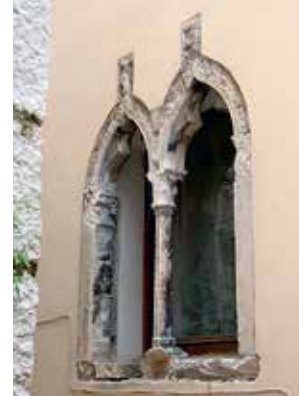
31 Projekt 41: bifora prije radova Project 41: bifora before restoration
