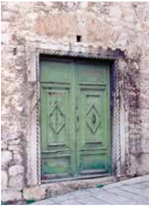
17 Projekt 19: stanje portala prije radova Project 19: condition of portal before restoration
