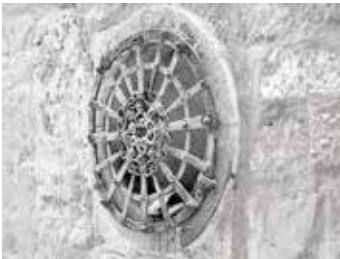
5 Projekt 7: stanje rešetke 1984. godine Project 7: condition of metal grating in 1984
