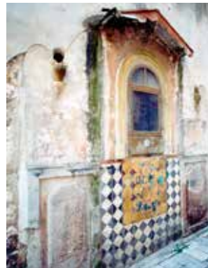
15 Projekt 18: stanje kapelice prije radova Project 18: condition of chapel before restoration
