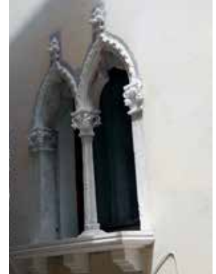
32 Projekt 41: bifora nakon radova Project 41: bifora after restoration
