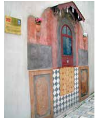
16 Projekt 18: stanje kapelice nakon radova Project 18: condition of chapel after restoration
