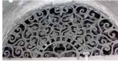
3 Projekt 2: stanje rešetke prije radova Project 2: condition of metal grating before restoration
