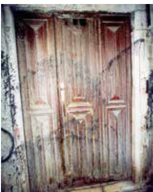
9 Projekt 10: stanje prije radova Project 10: condition before restoration
