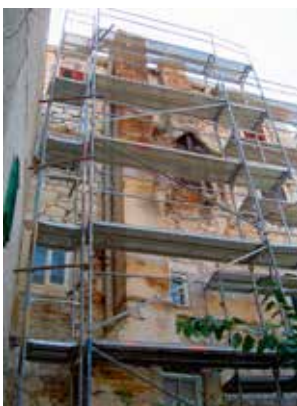
33 Projekt 44: stanje dimnjaka prije radova Project 44: condition of chimney before restoration
