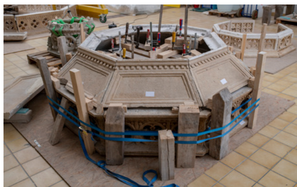
14. Split, radionica Odsjeka za kamenu plastiku, probna montaža drugog kata (fototeka HRZ-a, snimio J. Kliska, 2019.) Split, workshop of the Section for Stone Sculpture, trial installation of the second tier (HRZ Photo Archive; J. Kliska, 2019)
