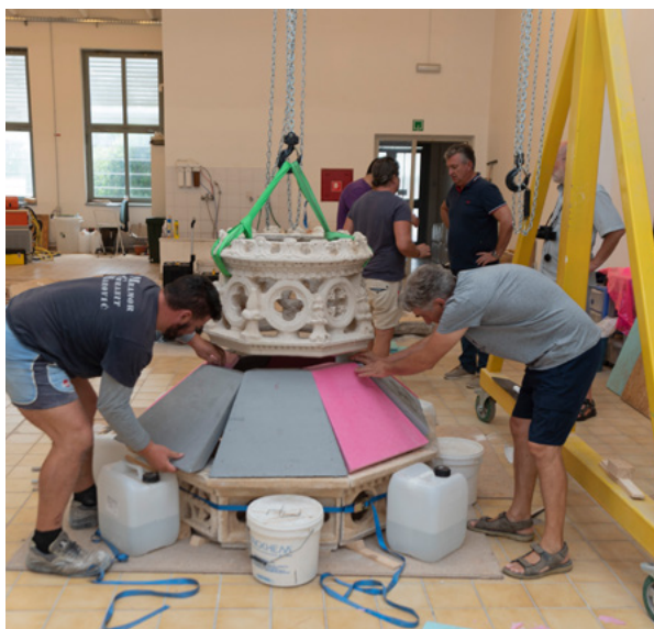
15. Split, radionica Odsjeka za kamenu plastiku, probna montaža s modelima F krovišta (fototeka HRZ-a, snimio P. Gamulin, 2019.) Split, workshop of the Section for Stone Sculpture, trial installation with F-roof models (HRZ Photo Archive; P. Gamulin, 2019)
