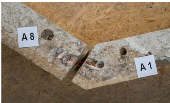
6. Dvostruke rupe od klamfi i trnova na gornjim ploham elementa A1 i A8 (fototeka HRZ-a, snimio J. Kliska, 2019.) Double holes made by clasps and thorns on the upper surfaces of elements A1 and A8 (HRZ Photo Archive; J. Kliska, 2019)
