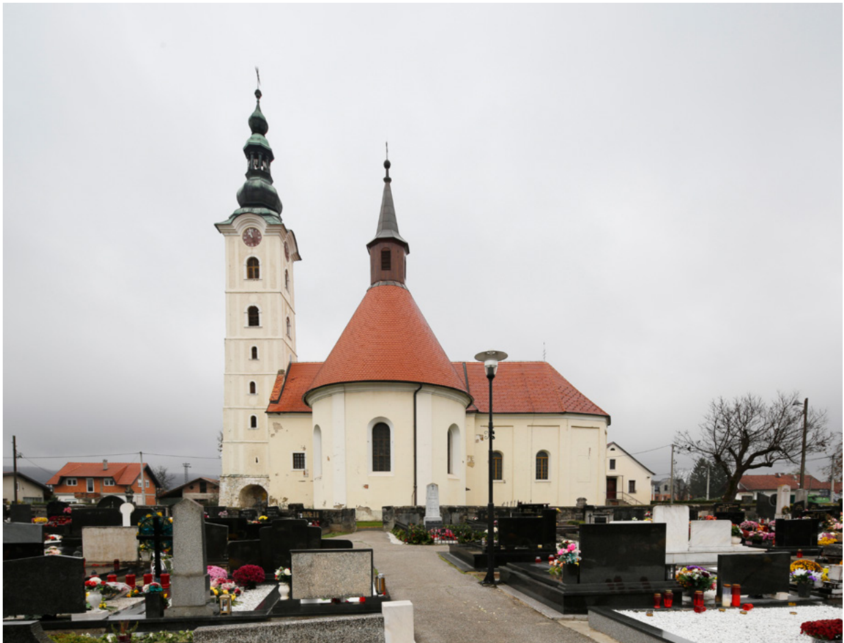
22. Brdovec, župna crkva sv. Vida, pogled na južno pročelje s kapelom sv. Barbare (MKM, KO ZG – F, snimio Z. Bogdanović, 2020.) Brdovec, parish church of St. Vitus, view of the southern façade with the chapel of St. Barbara (MKM, KO ZG – F; Z. Bogdanović, 2020)
