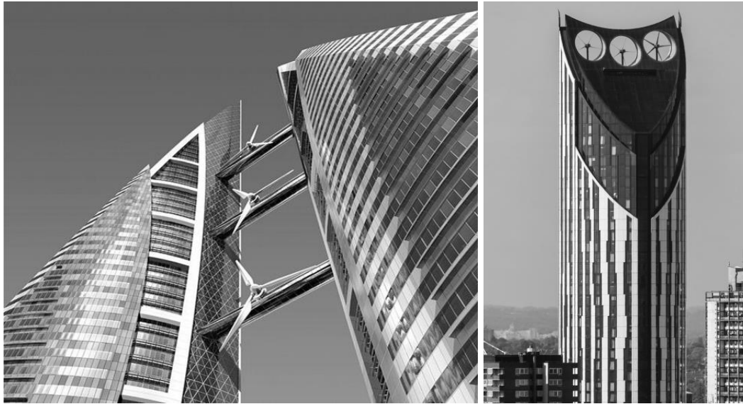
Figure 2. Wind turbines mounted on buildings. A) World Trade Center in Bahrain [5] b) Strata SE1 Tower [6].
