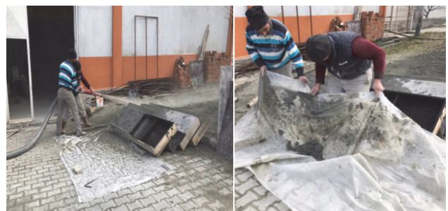
Figure 4 Shotcrete application and collecting the rebound material
