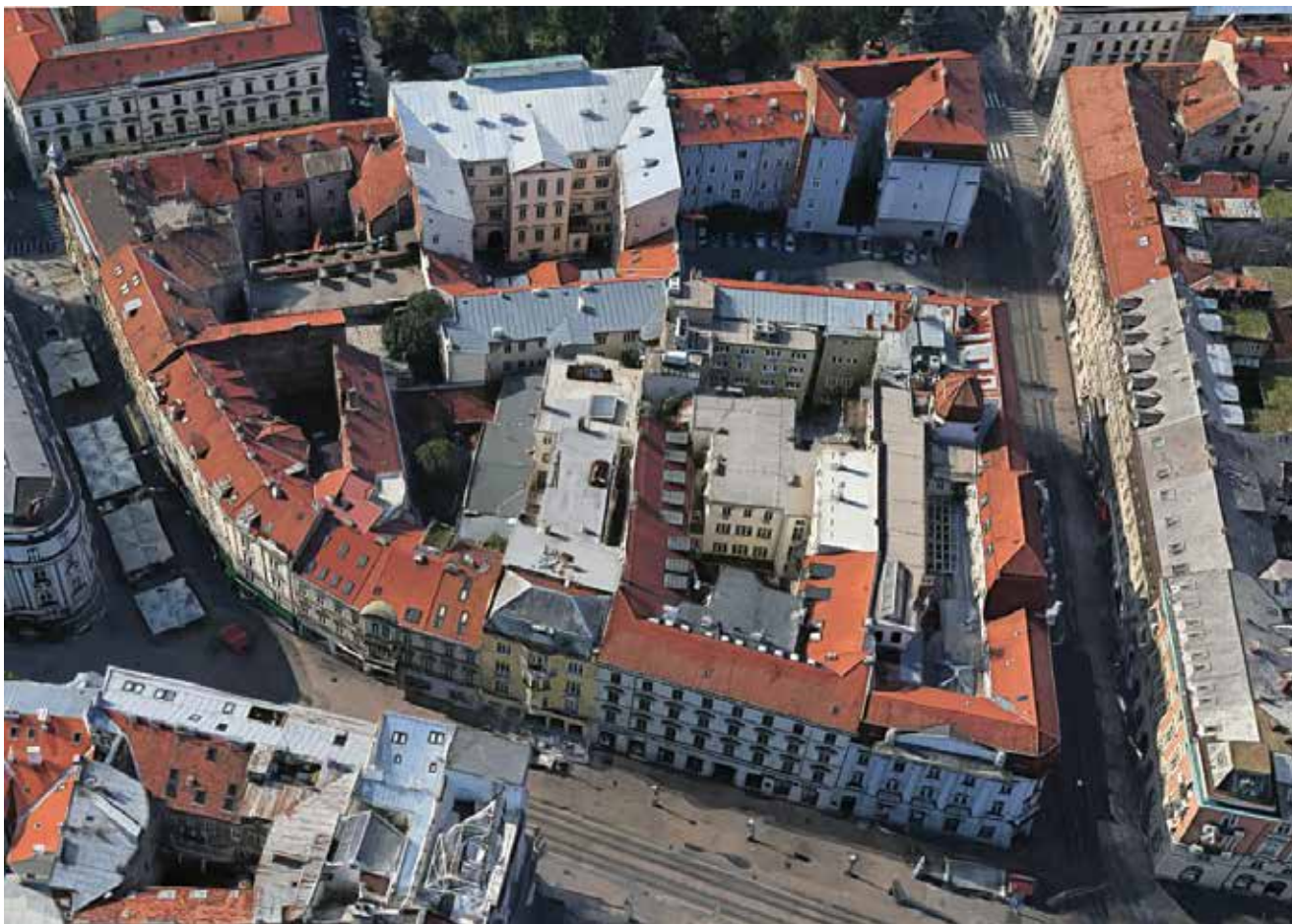
1. Zračna snimka bloka < https://www.google.hr/maps/ > Aerial view of the block
