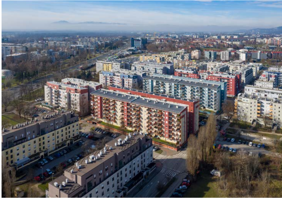
Program društveno poticane stanogradnje (POS) u Španskom u Zagrebu, 2020. Foto: Paolo Mofardin / State-Subsidized Housing Construction (POS) in Špansko in Zagreb, 2020. Photo: Paolo Mofardin ← ↑ ↓
