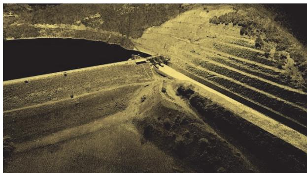
Figure 5 Point cloud of the scanned dam with a spillway
