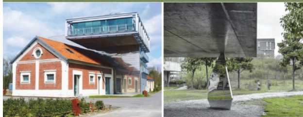
Figure 13 Glazed hovering extension, Pas-de-Calais, France, 2014 (Hérault Arnod Architectes) /inhabitat.com/ and Blossom Pavilion, Shanghai, China, 2015 (Atelier Deshaus) /archdaily.com/
