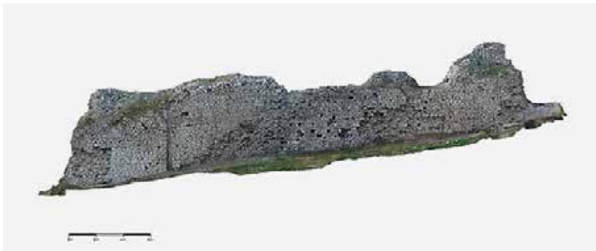
Sl. 3. Ortofotografija unutarnjeg lica zapadnog zida utvrde (izradio: LupercalMT j.d.o.o.) Fig. 3 Orthophoto image of the west wall inner face in the fort (made by: LupercalMT j.d.o.o.)
