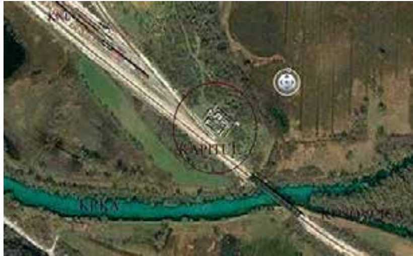
Sl. 4. Pogled na Kapitul i talijansku vojarnu nakon uklanjanja raslinja 2011. godine (izvor: Google Earth) Fig. 4 View of Kapitul and the Italian barracks after the removal of the vegetation in 2011 (courtesy of Google Earth)
