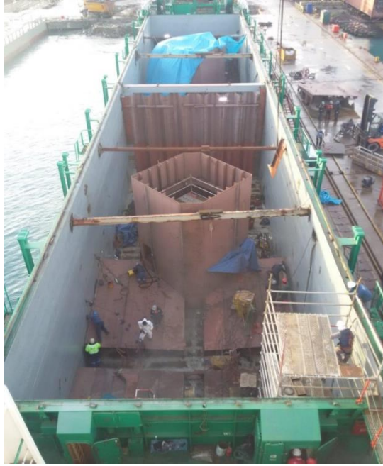
Figure 2 Ship no.1 cargo area photo taken in the shipyard during major conversion and new parts installation into existing hull
