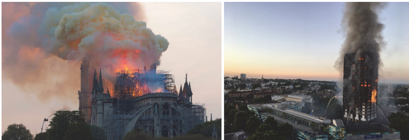
Slika 2. Notre Dame u požaru [6], Grenfell Tower u požaru [7]
