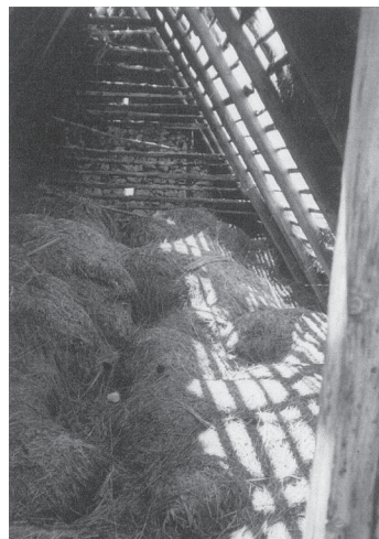
FG. 13. Attic of a shed with a pitched roof
