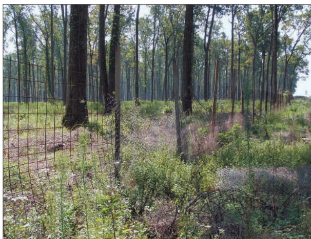
Slika 7. Segment ograde od armaturne mreže zbog oštećenja privremeno zamijenjen pletenom žicom. Figure 7 Armature net protective fence segment temporarily replaced with wire network.
