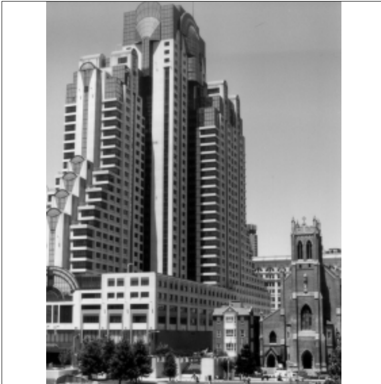
FG. 10. Preserving the sense of time: the architectural form of Merriot hotel trying to emulate the form of St. Patrick's church in San Francisco.
