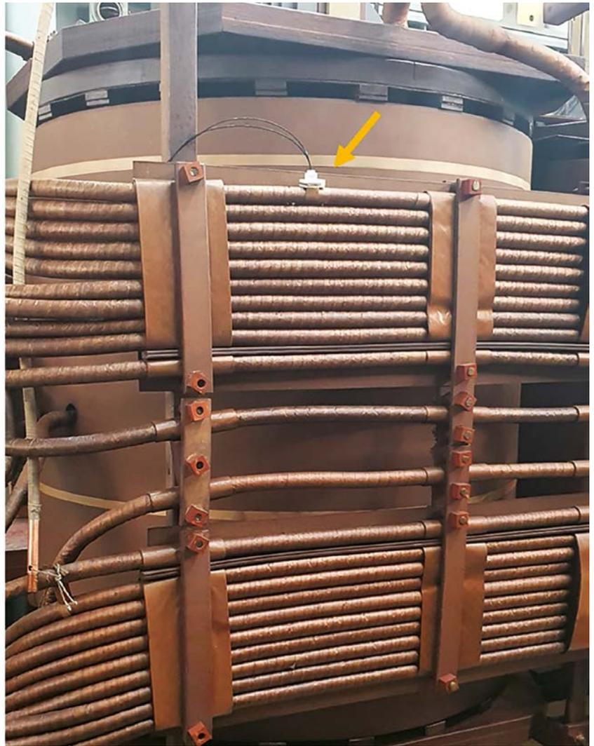
Figure 14. Sensor head for monitoring insulation paper mounted on a lead inside the transformer
