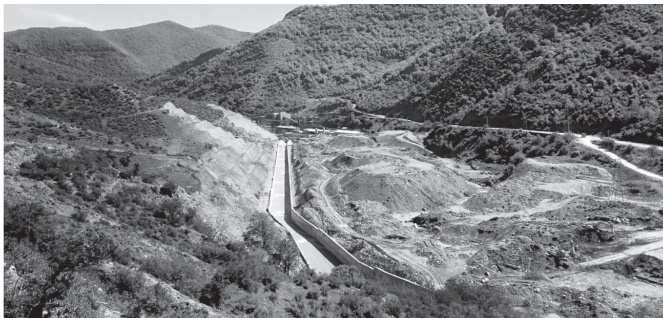
Fig. 1 Alborz Markazi coal washing plant in forest area
