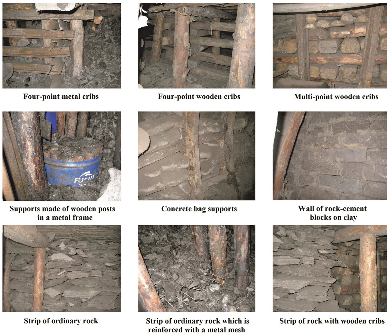
Figure 2: Photos of artificial constructions for the protection of mine roadways
