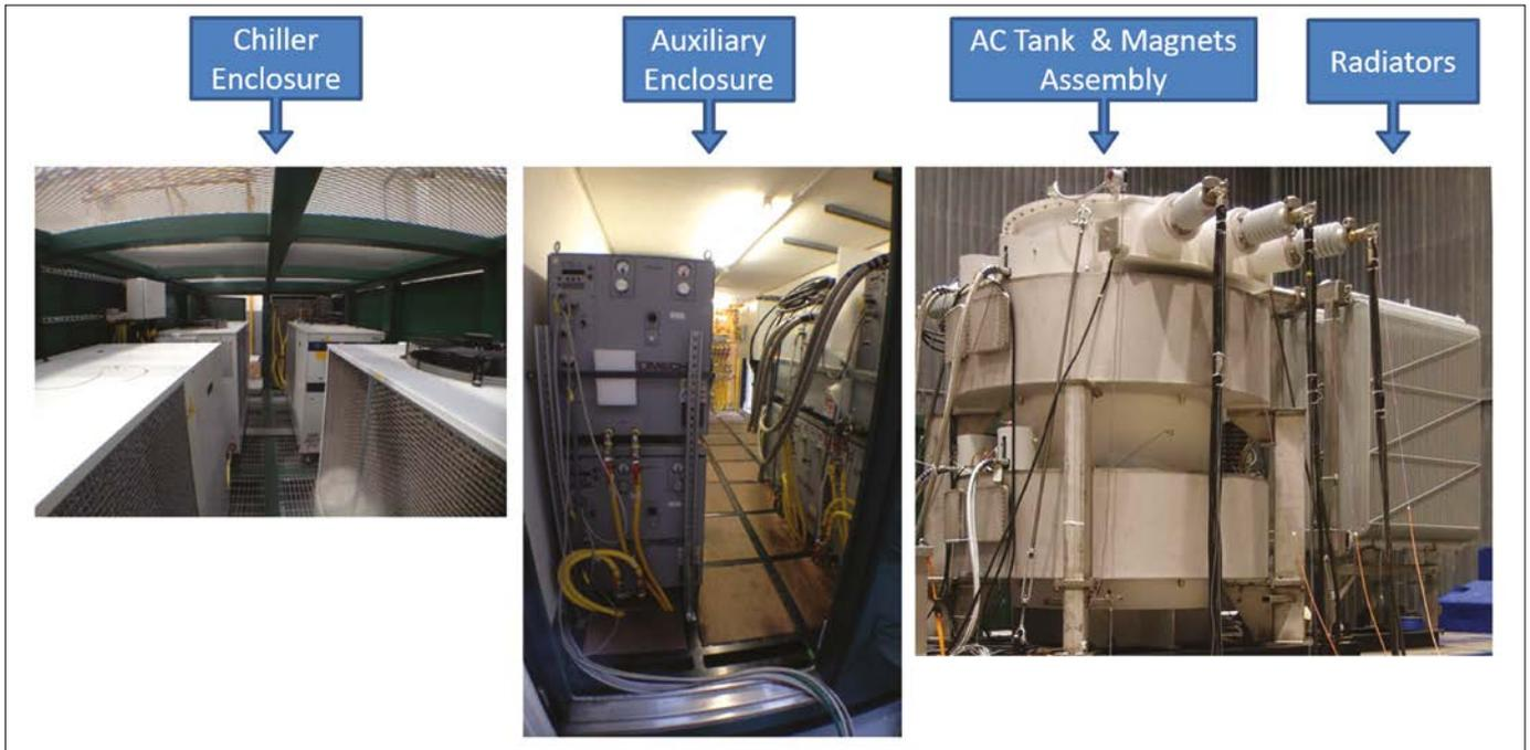
Figure 10. L-R chiller enclosure, auxiliary enclosure and reactor tank / magnets / radiators assembly
