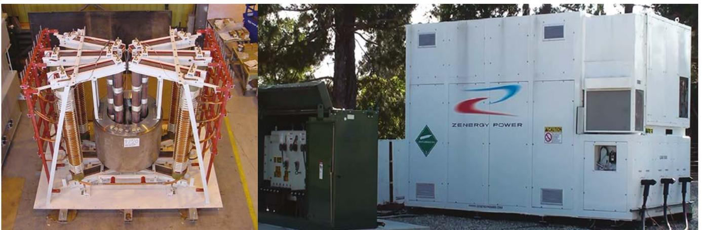
Figure 1. Closed-core arrangement showing active parts (left) and installed device (right)
