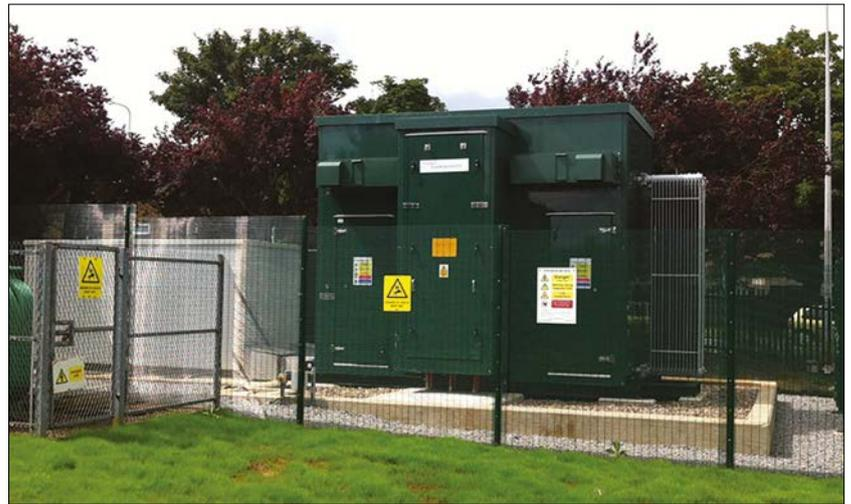
Figure 4. 11 kV; 1250 A open-core FCL installed in the primary substation
