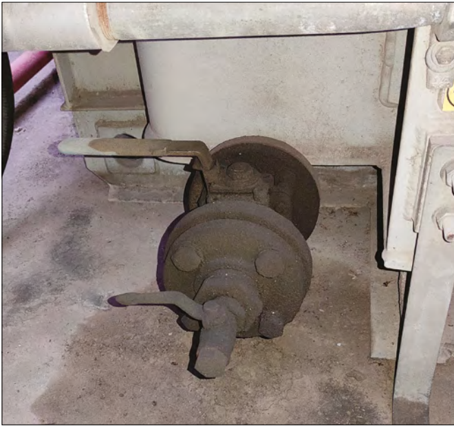
Figure 8. Examples of 2 valves assembly of sampling valves.
