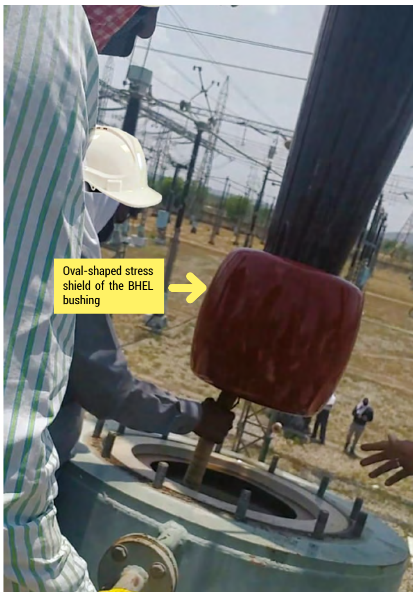
Figure 1. The process of removing the 420 kV BHEL bushing with the Hydra crane.
