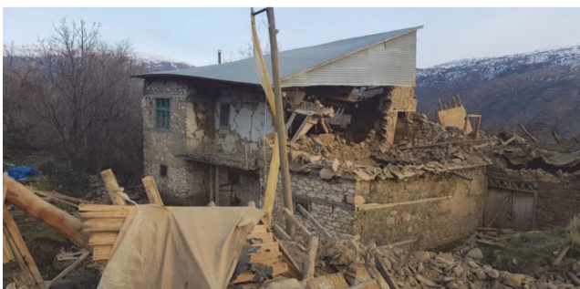
Figure 25. Collapsed masonry building in lower Cevrimtaş village (building 4)
