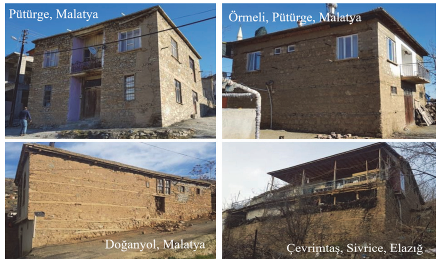
Figure 13. Typical masonry buildings constructed in the region
