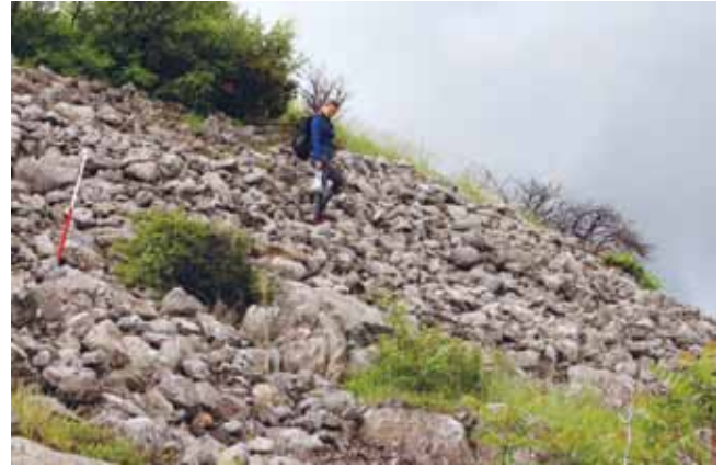
FIGURE 7. Remains of the collapsed ramparts on the north and northeast sides between Velika Orišnica and the Petrovac hill (photo by Ž. Miletić).
