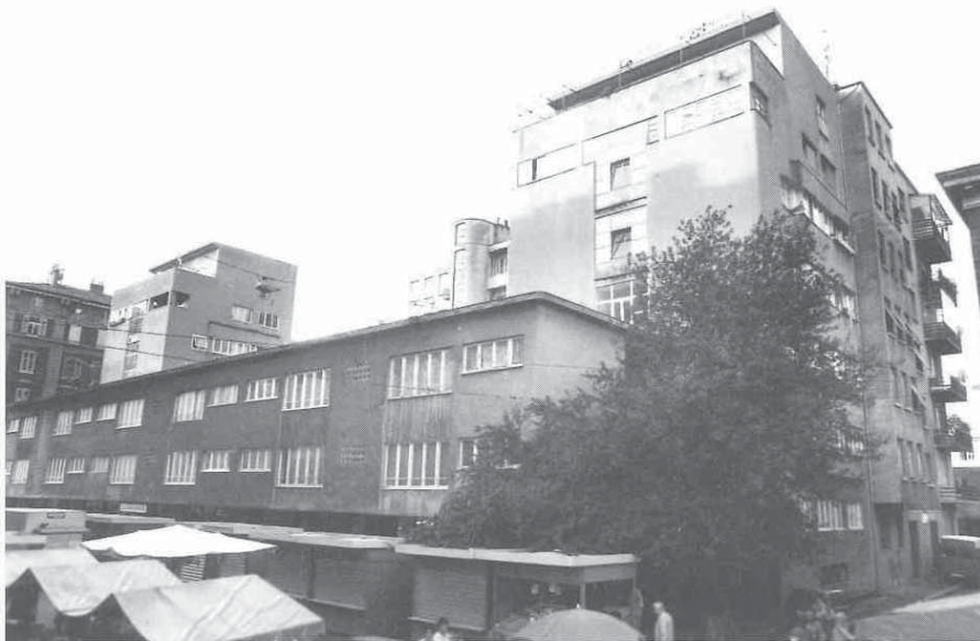
6 Hinko Bauer, Stambena zgrada, 1951. / Hinko Bauer, Apartment Building, 1951
