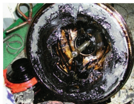
Fig. 6 Accumulations of asphalt components in the purifier bowl
