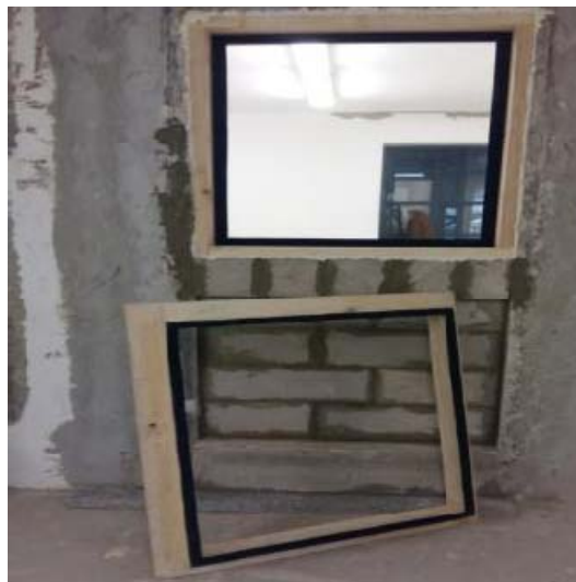
Figure 2. Installation of soundproof panels during the experiment
