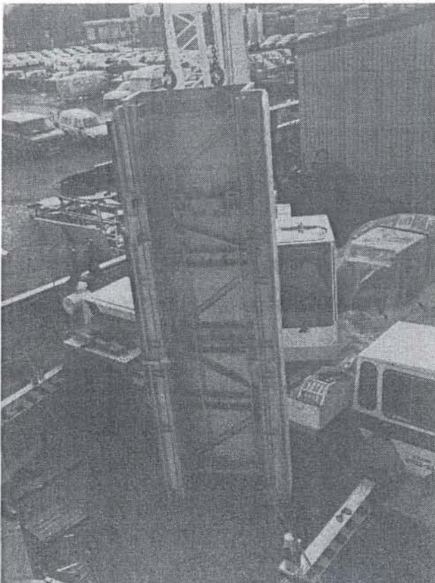
Fig. 10: Canary Wharf FC5 London. Plaza level – column cladding, steel frame back view. To be noticed the scheme of diagonal reinforcements to avoid stresses on stone sheets.
