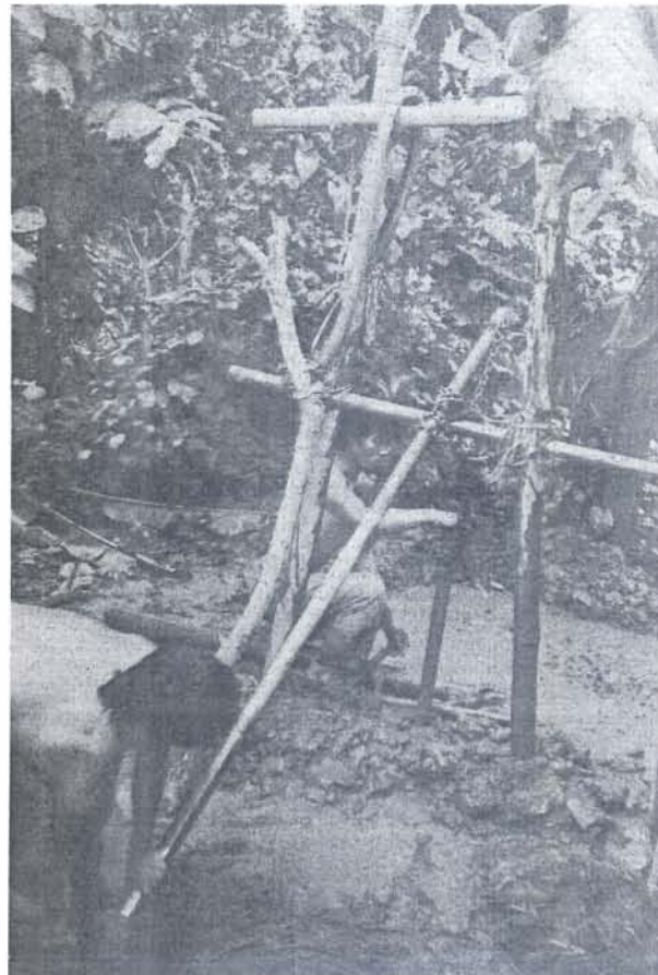
Fig. 2 Sludger drilling rig
