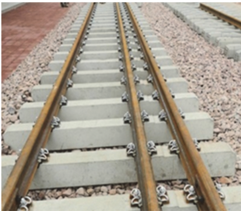
Figure 3 Physical dual-gauge railway
