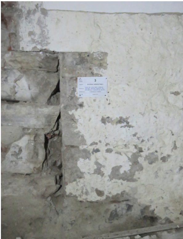
5. Dvorac Kerestinec, spoj najstarije zidane strukture s dograđenom sjeverozapadnom kulom (snimka: V. Jakaša Borić) Kerestinec castle, a combination of the oldest masonry structure with an extended northwest tower (V. Jakaša Borić)
