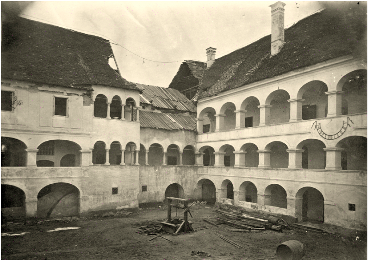
7. Dvorac Kerestinec, dvorišna pročelja zapadnog i sjevernog krila (MKM-FKB, snimka: I. Standl, 1880.) Kerestinec castle, courtyard façade of the west and north wings (MKM, FKB, I. Standl, 1880)
