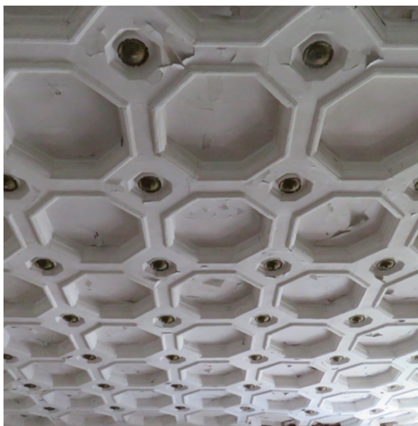
17. Kasetirani strop glavne dvorane zapadnog krila dvorca Kerestinec (snimka: V. Jakaša Borić, 2019.) Coffered ceiling in the main hall of the west wing of Kerestinec castle (V. Jakaša Borić, 2019)
