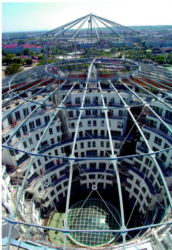
3. Gasometer complex in Vienna, interior of Gasometer C ( https://www.wehdorn.at/projects/gasometer/ , 17/08/2021) Kompleks plinomjera u Beču, unutrašnjost plinomjera C ( https://www.wehdorn.at/projects/gasometer/ , 17. 8. 2021.)
