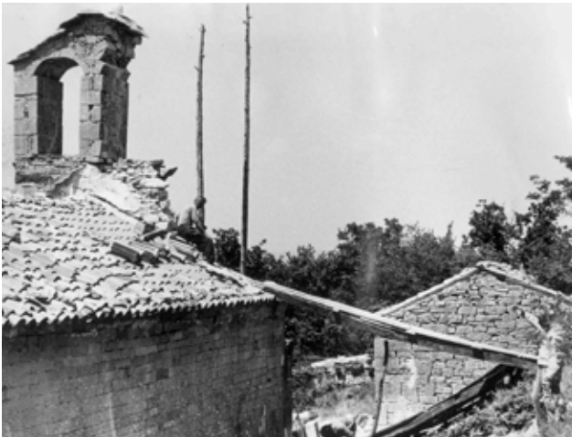
11 Obnova urušene preslice 1972. (foto: Ružić, fototeka KORi, 1972.) Restoration of damaged bell-gable in 1972 (photo: Ružić, KORi photo library, 1972)
