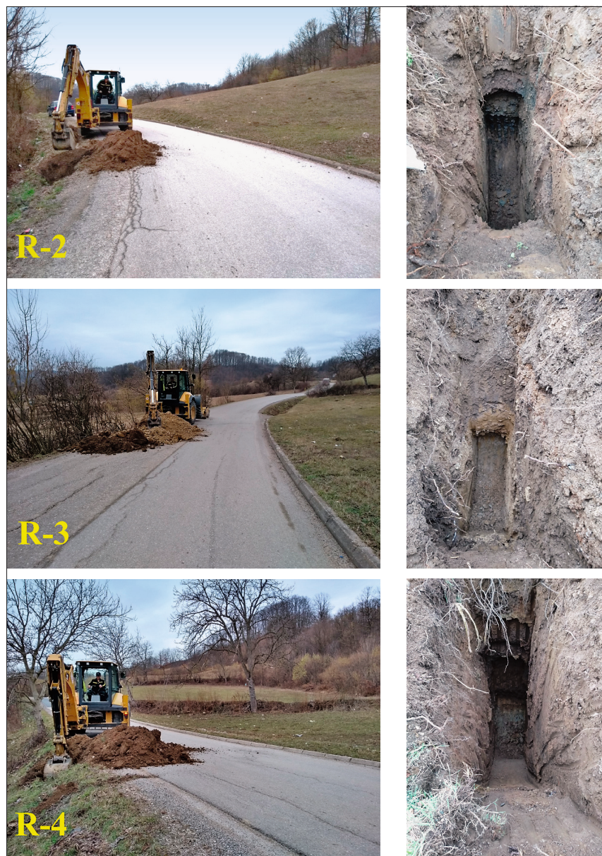
Figure 6: Exploration excavations R-2, R-3 and R-4
