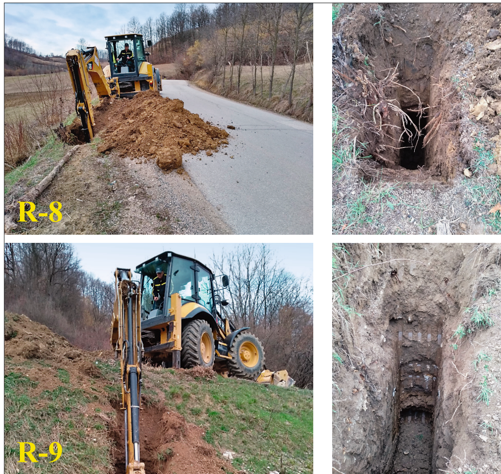
Figure 8: Exploration excavations R-8 and R-9
