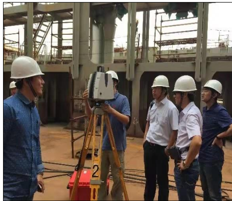
Fig. 1 Scanning the cell guide of container ship
